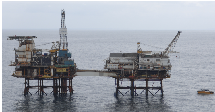
Figure 5: Aerial photograph of Beatrice 11/30-A consisting of two bridge-linked platforms. Height 86m. Acquired 14th April 2016.
