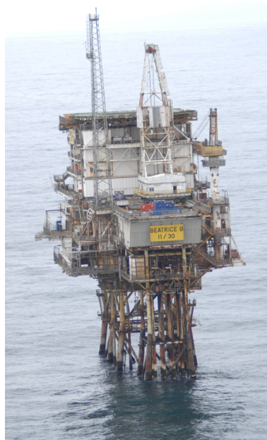
Figure 6: Aerial photograph of Beatrice 11/30-B platform. Height 82m. Acquired 14th April 2016.
