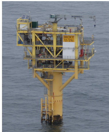
Figure 9: Aerial photograph of Jacky 12/21c platform. Height 34m. Acquired 14th April 2016.
